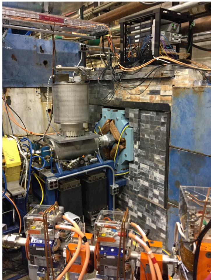
Figure 2.8-8: The beam-stop line and lead-brick shielding wall.
